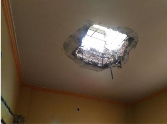
*Fig 1: Demolition of Slab on Site*
