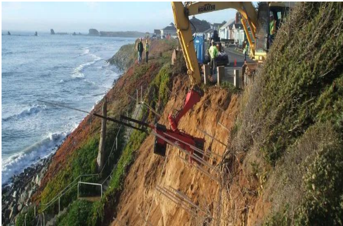
Fig.5: Launched soil nail method
