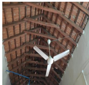
Fig 3: Mangalore tiles roofing with truss
