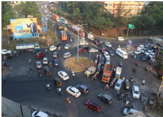
Fig. 1: Aerial view of Nanthoor Intersection
