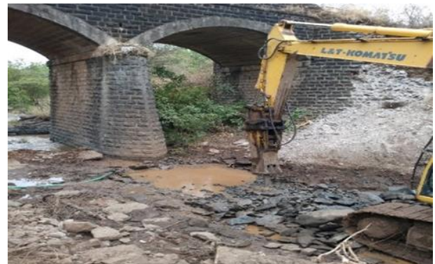
Fig.5.2.1: Excavation for foundation
