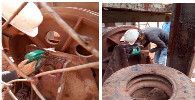
Fig No. 6 Structural Cracks in Beam BC
