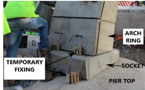
Fig.5.2.4 Socket placed on pier top
