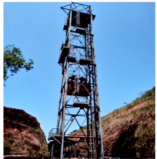
Fig. 1 Gravity Tension Tower
