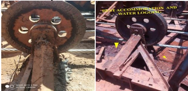
Fig No. 2 Structural Cracks in Beam BC
