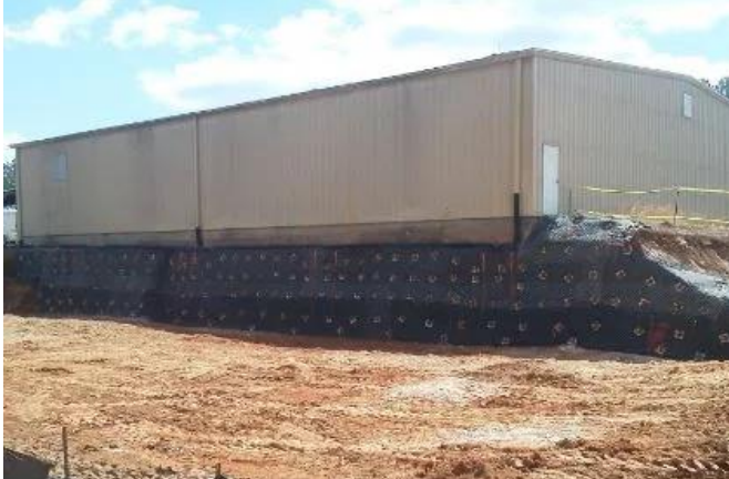
Fig.2: Driven soil nail method
