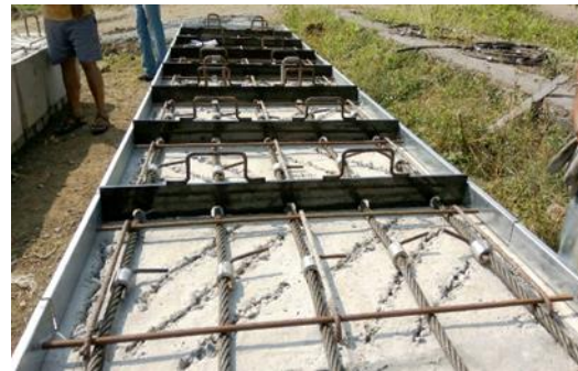
Fig.5.1.6: Wire rope placed on Blocks
