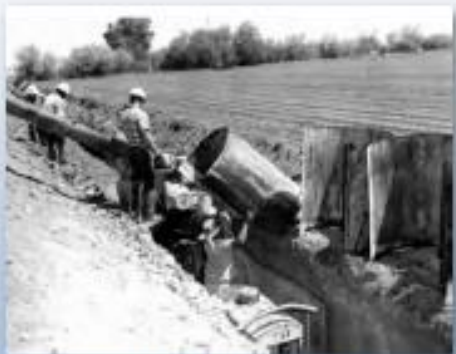
Cast-in-place concrete pipe Arizona, USA. 1963
