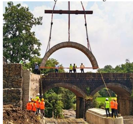
Fig.5.2.5 Full Lift of Arch Strip
