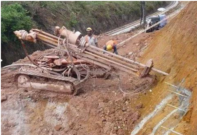
Fig.1: Drilled and grouted soil nailing method
