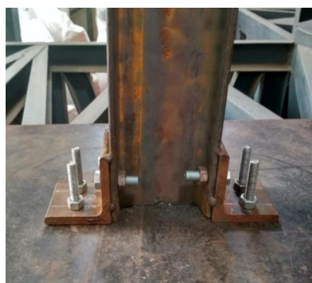
Fig.3 Bolted Connection in the base of column
