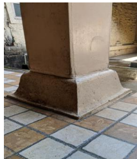
Fig 13. Wooden column with Stone support
