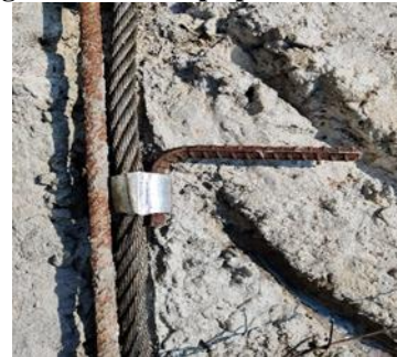
Fig.5.1.7: Ferrules and Rod
