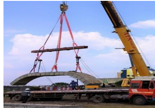
Fig.5.1.10 Half lift of arch strip
