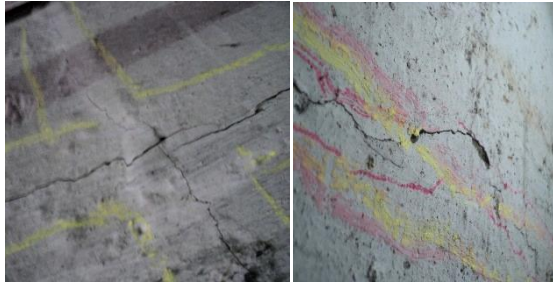
Fig. 4: Structural Cracks Beam DE
