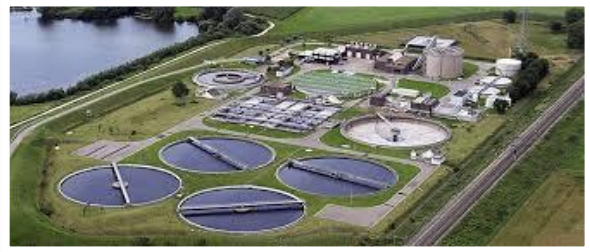
Fig no :-1 Sewage treatment plant
