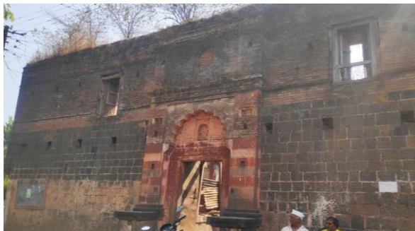
Fig 10: Façade of Kore Wada
