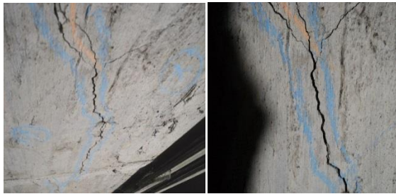
Fig. 5: Structural Cracks at Col.- Beam BA-AF Junction
