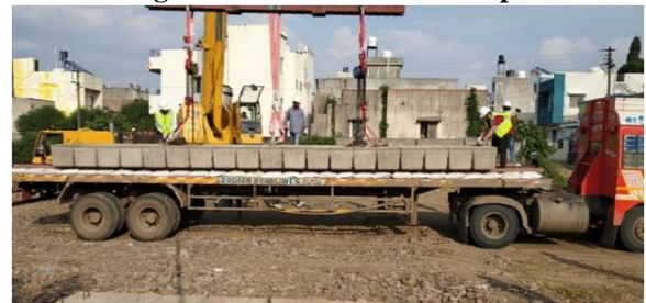
Fig.5.1.11 Arch Strip placed on trailer for transportation
