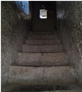
Fig. 12 one of the staircases
