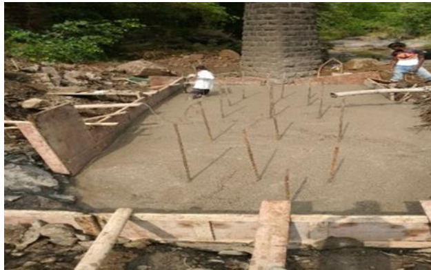
Fig.5.2.2 Cat-in-situ of foundation
