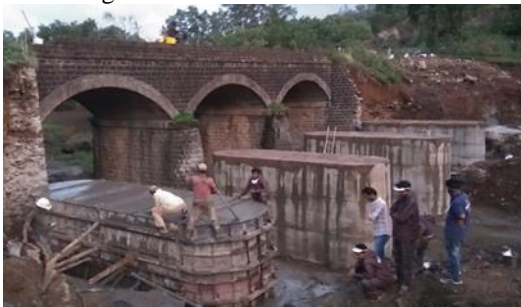
Fig.5.2.3 Cast-in-situ pier and abutment
