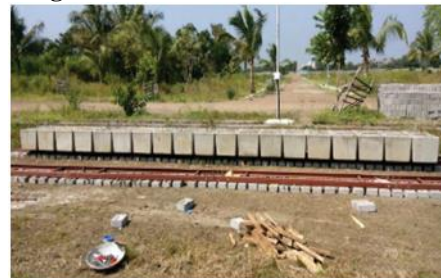
Fig.5.1.3: Blocks arranged line and leveling
