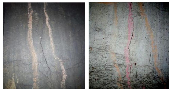
Fig. 3: Structural Cracks in Beam BC
