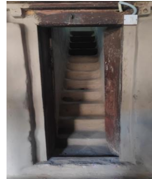
Fig 12: one of the staircase
