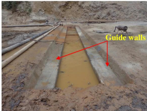
Figure-5: Photograph showing guide walls along the panel trench
