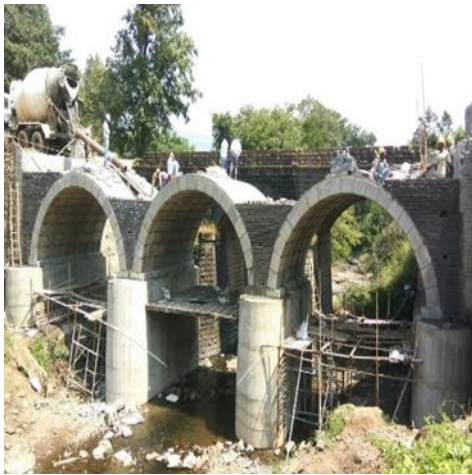
Fig.5.2.6 Spandrel wall and Plum filling
