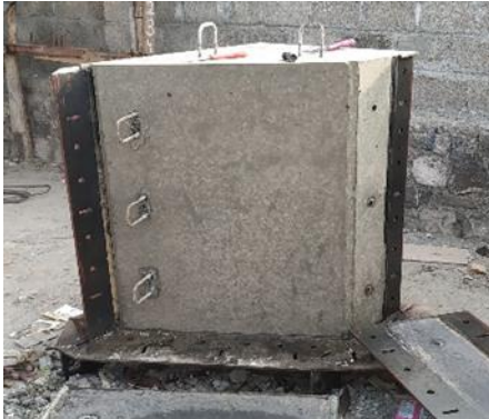
Fig.5.1.4 Precast PCC Socket
