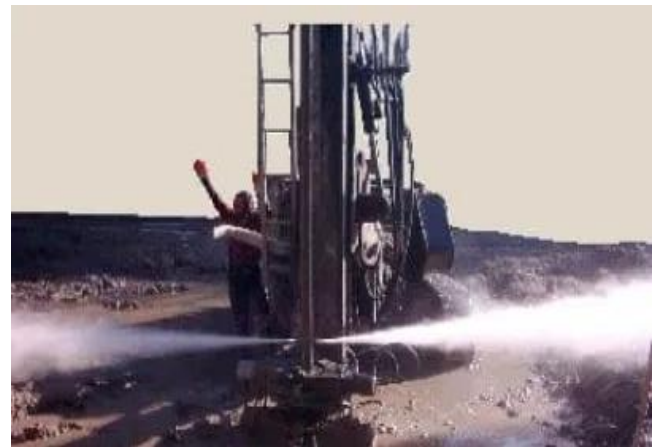
Fig.4: Jet grouting soil nail method
