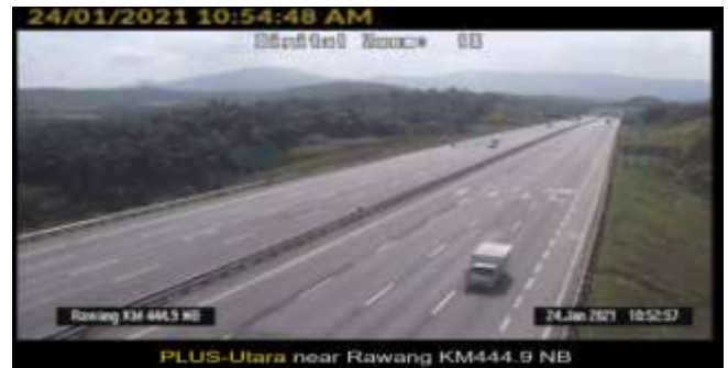
Fig.1 Example of CCTV view
