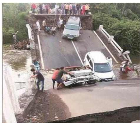
Fig 1: Gujarat: Seven injured as bridge collapses on Junagadh-Sasan highway
