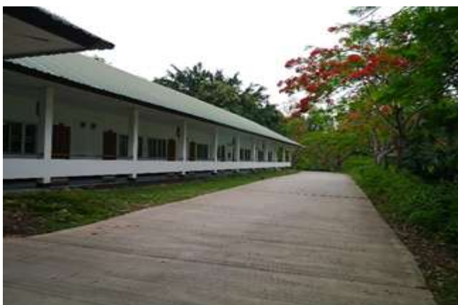
Fig.4 The guest room building of Phayao university hotel
