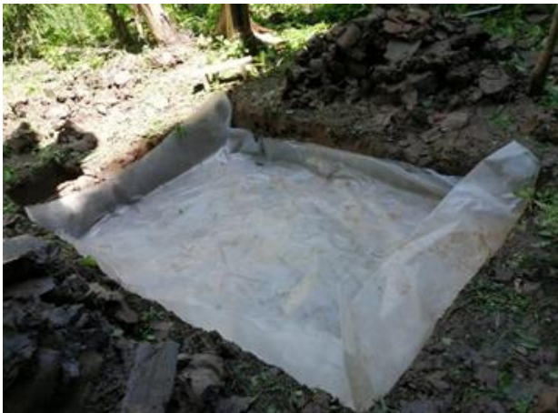
Fig. 2 Lay the plastic sheet on the ground plot
