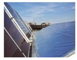
Fig. 3: Silver sheet reflection on solar panel
