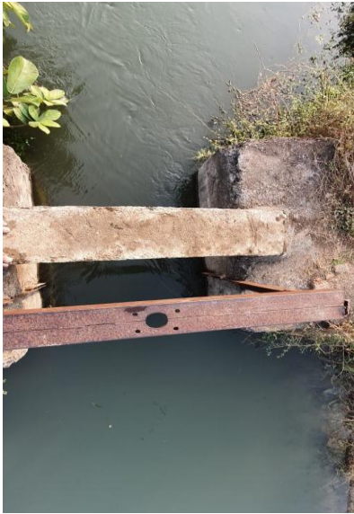
Fig. 6. Top View of Canal
